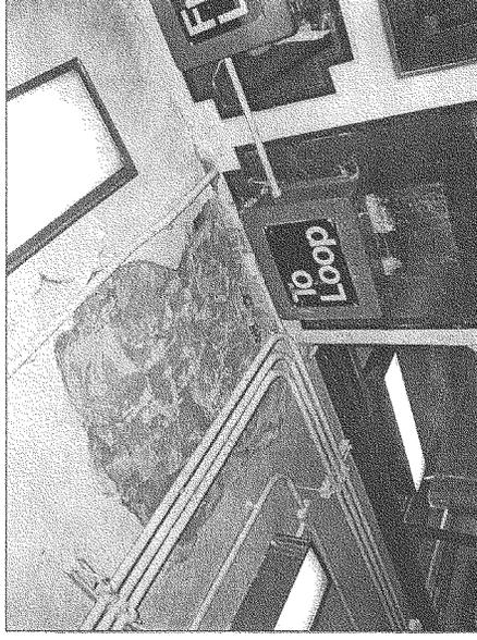
Ceiling damage in station roof which provides the structural support for the track above
