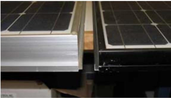
**Figure 31: Examples of external flange frames**
