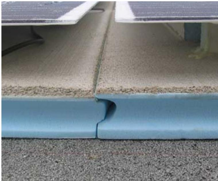
**Figure 56: PowerGuard tile with reduced coating thickness (on right)**
