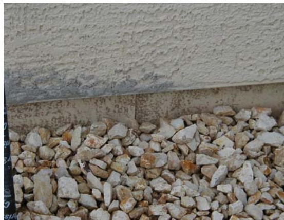
Figure 32. Edge insulation properly protected with sheet metal
