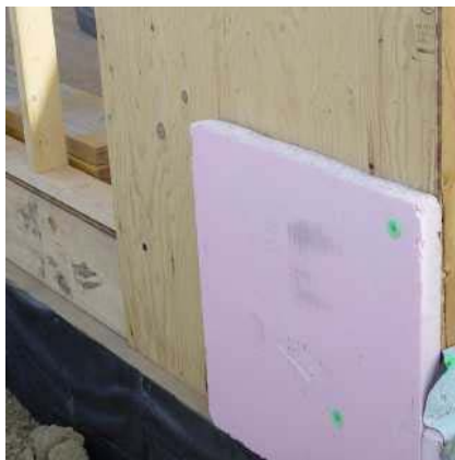
Figure 28. The houses feature 1-1/2-in. XPS foam at corners
