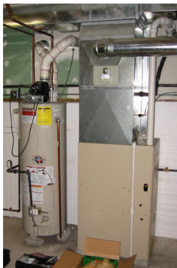
Figure 43. Sealed-combustion furnace and water heater in the first home.
