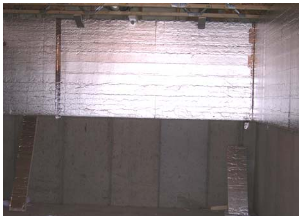
Figure 38. Foil-faced polyisocyanurate insulation
