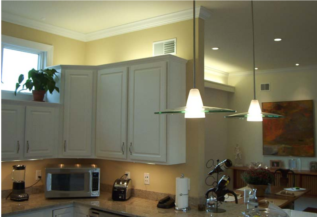
Figure 46. Over-cabinet (fluorescent) and under-cabinet (halogen) lighting was used at the Kacin Construction project. Cove lighting, consisting of strip fluorescent lamps and recessed downlights with CFLs, were used in the adjacent dining room.
