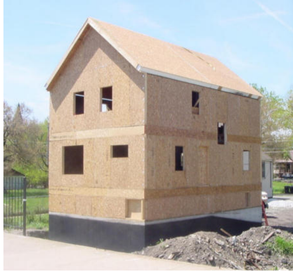
Figure 42. SIPs installed in the first home
