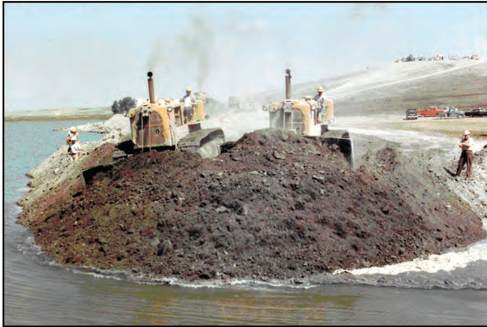
Closure of Big Bend Dam in 1963. Construction of six large reservoirs on the upper Missouri River have greatly decreased the amount of suspended sediment and turbidity in the lower river. (Photograph courtesy of the U.S. Army Corps of Engineers.)
