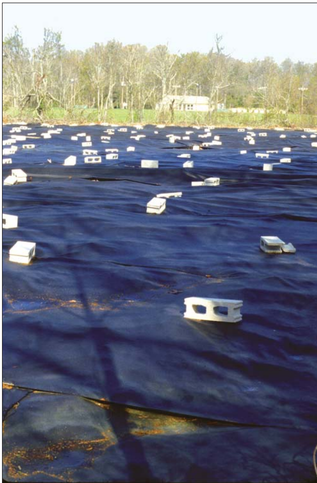
Figure 4. "Drop zone" of high-density pellets covered with geotextile fabric to protect waterfowl and other birds. (Cinder blocks keep the fabric from blowing away. The white building in the background is Broadkill Sportsman's Club house.)
