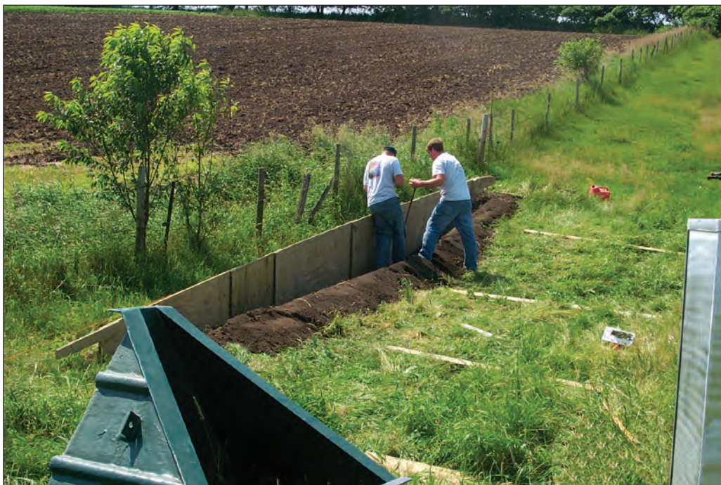
Figure 5. Plywood wingwalls were used at most edge-of-field stations to provide a flume-mounting surface and to direct all surface-water runoff through the flume.
